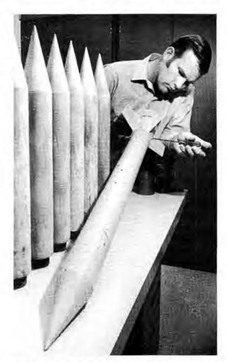
JACK KIKER (9327) assembles Sandia Ice Penetrometer (SIP) planned for use during Coast Guard-sponsored tests in Greenland and northeast Canada in mid-April.
